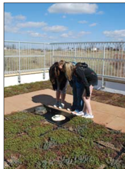
Bowling Middle School (Owen County) eighth-graders, from left, Elizabeth Stewart, Autumn Gover and Kaylee Boling, examine the details of the new school's vegetative roof — only the second for a Kentucky school. The roof is designed to be both environmentally sound and a learning space ... Article on Page 10.
